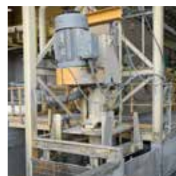
Below: Warman® SPR pump in coal sump application.
