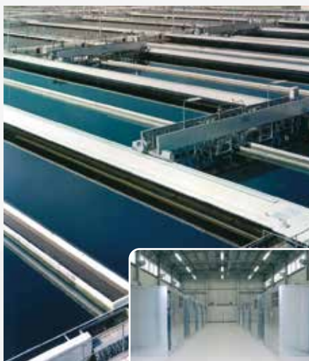
• Sewage purification: ROBOX evolution blower unit
