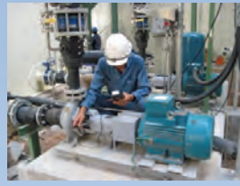
Site test & commissioning work
