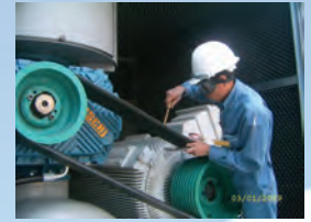
Belts tensioning set up
