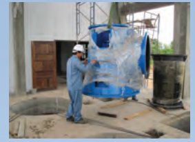
Pump installation service
