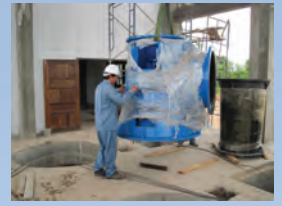
Pump installation service
