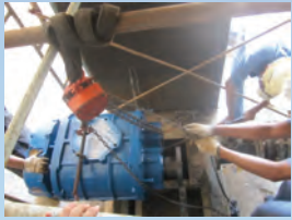
Pump installation service
