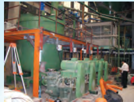
Pump's inspection Service
