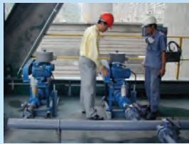
Site inspection service
