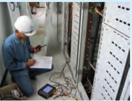
Electrical testing work
