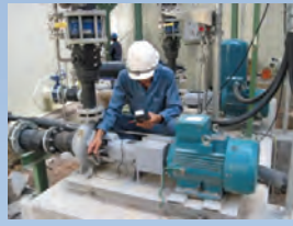
Site test & commissioning work
