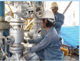
Site inspection service
